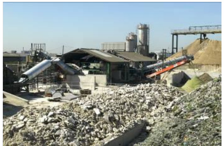
View of C&D site
