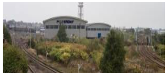
Powerday facility under construction
